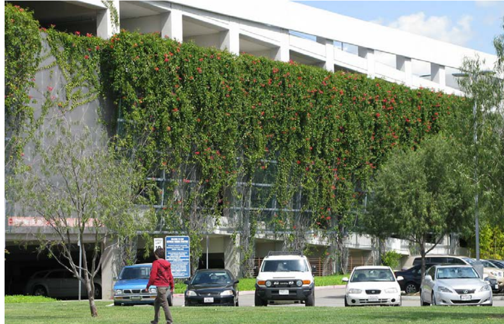
A GREEN SCREEN ON A PARKING STRUCTURE PROVIDES VINES WITH A SUPPORT ON WHICH TO GROW. WHEN MATURE, THE VINES HELP SCREEN THE PARKING STRUCTURE FROM VIEW.
