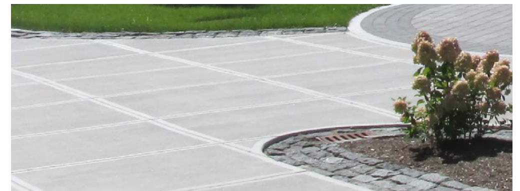
GRANITE COBBLE GUTTERS ALONG SIDEWALKS PROTECT LAWN AND PLANTINGS FROM WINTER PLOWING AND SALT DAMAGE
